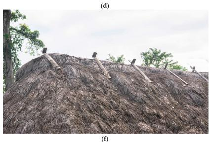
**Figure 8.** Supplementary illustration relating to construction processes, (**a**) Weaving with *teren* leaves, (**b**) Roof finishing, (**c**) Detail of joint with vine ties, (**d**) Roof weaving, (**e**) Preparation of leaves for placing the ridge cap, (**f**) Ridge cap fastening with bamboo (Source: Author).
