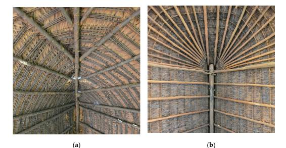
**Figure 10.** Types of structure and weaving, (**a**) Structure with single support in herringbone, with *"teren"* leaf weaving arranged horizontally, (**b**) Structure with two supports and hanging beams, with *"kampanak"* leaf weaving arranged vertically. (Source: Author).
